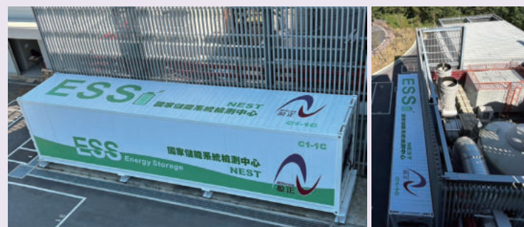
Tongliao Industrial Park - National Energy Storage System Testing Center
